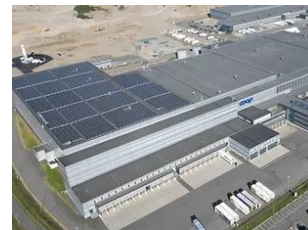
Clog warehouse: Design for a total of 3.7 MWp on rooftop and facade
