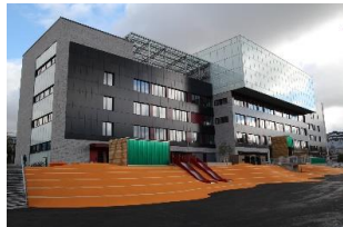
Brynseng school: BIPV facade: design, procurement and construction supervision
